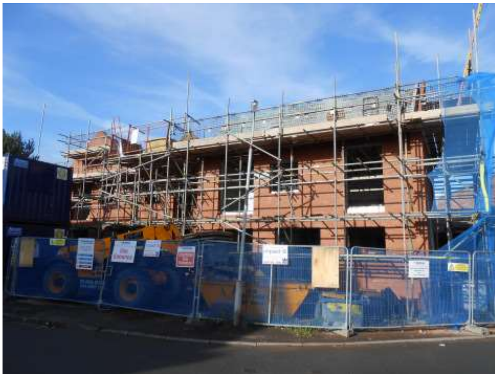
Figura 2 - Houses under construction on Birkenhead, Merseyside, England
